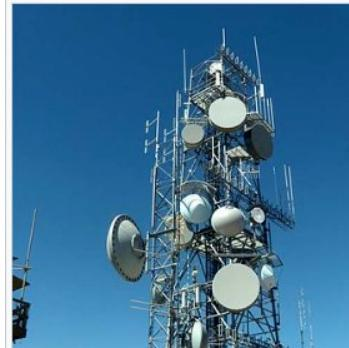
It is often used for point-to-point communication links over long distances, such as in microwave relay systems and satellite communication.
